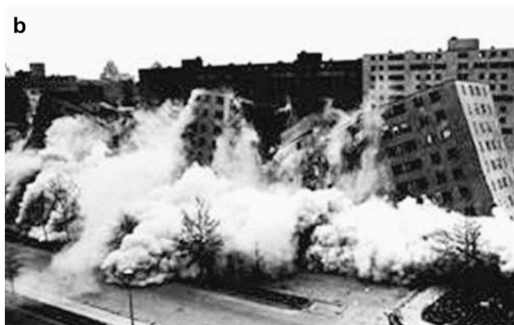
Figure 1 Demolition of Pruitt-Igoe housing project (© Newman, 1996)
